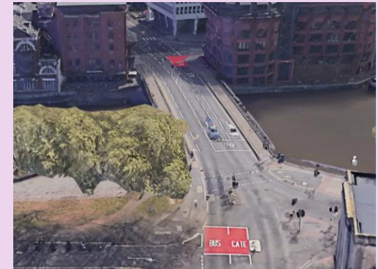
Bristol Bridge Bus Gate, with painted road surface 4
