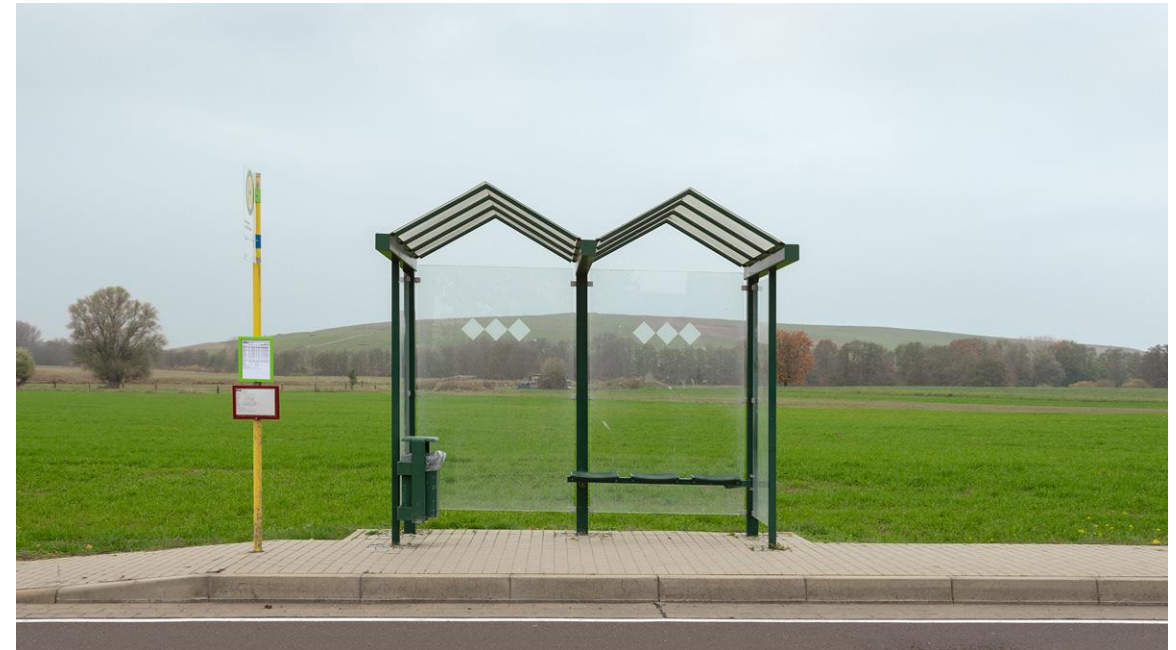
Rural bus stop in Germany, with shelter, clear and consistent branding, and timetables.
