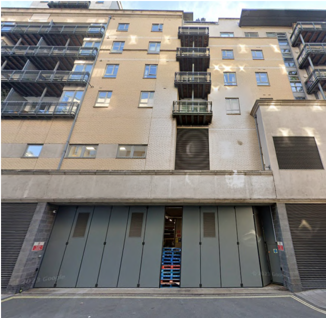
Figure 2-1 Supermarket loading bay in Pimlico, London – loading bay below residential bedrooms
