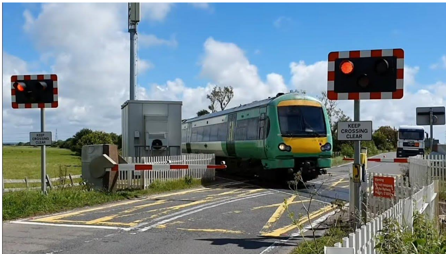
Figure 2.29: Star Level Crossing (A259/Marshlink Railway)
